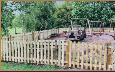
Our brand new park fence
