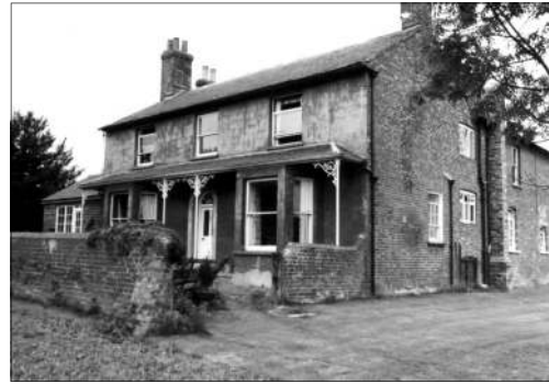
Lower Farmhouse, Brook Street, 1992
