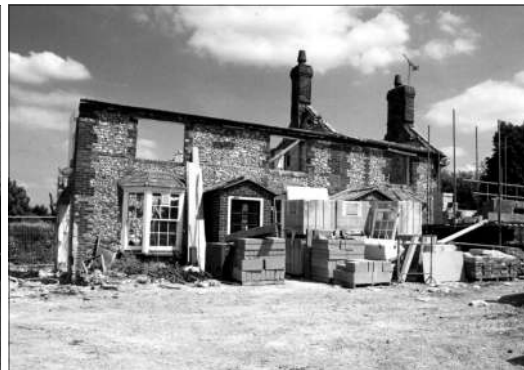
'Conversion' of The Shoulder to houses
