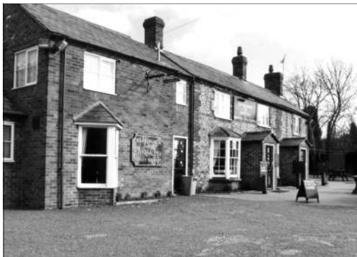
Shoulder of Mutton after extensions
