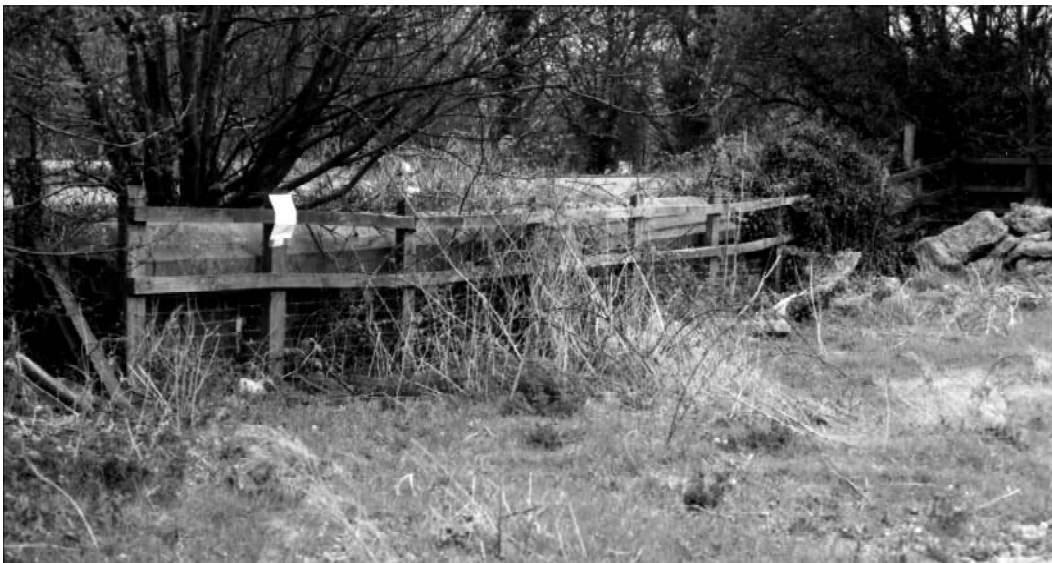
All that remains of the bridge on Aston Hill
