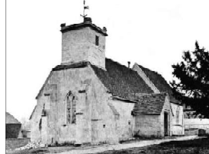
After repairs in 1830s
